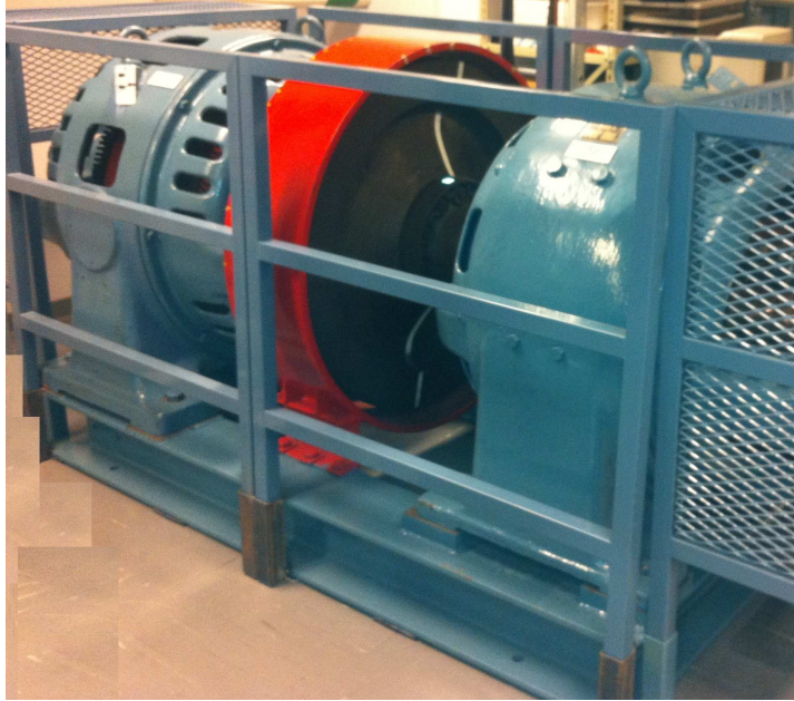
Fig. 7.3 Photo of the generator system comprising of the synchronous generator to the left end, the DC motor to the right end and the flywheel in between.
