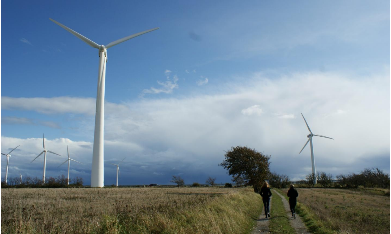
FIGURE 22: A PART OF THE WIND POWER PLANT AREA NÄSUDDEN, SEPTEMBER 2009.
