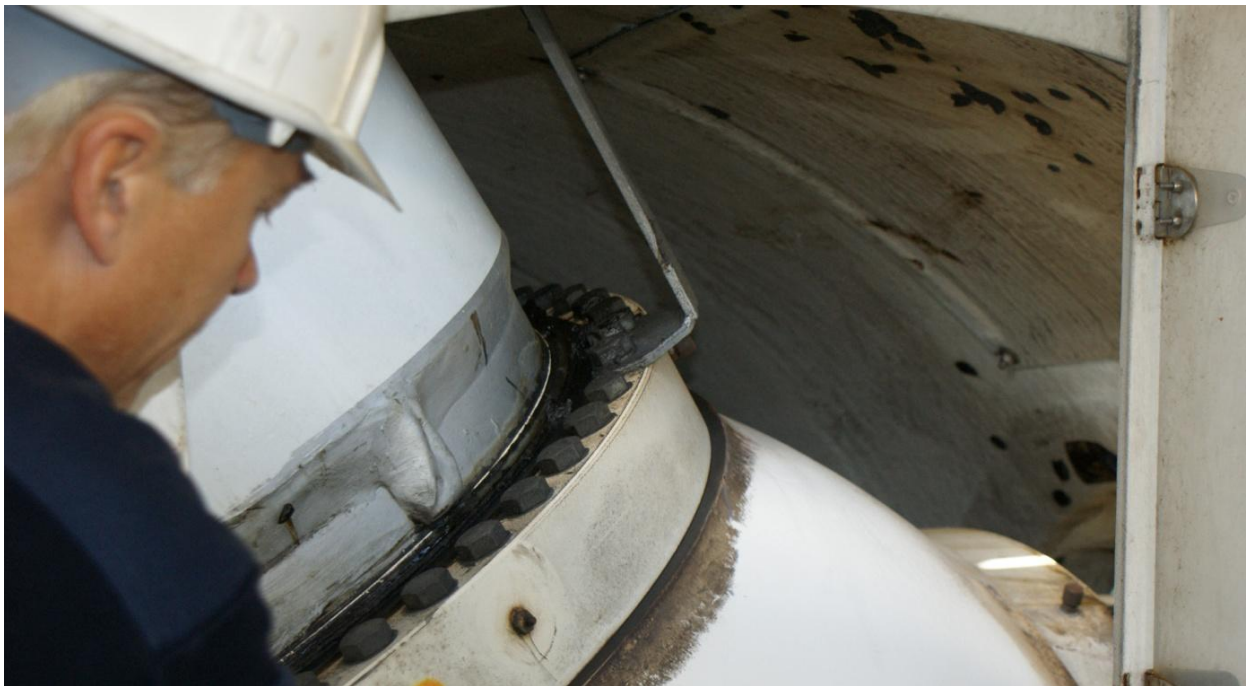
FIGURE 32: PHOTO TAKEN INSIDE THE MACHINERY OF A PITCH CONTROLLED WIND POWER PLANT.
