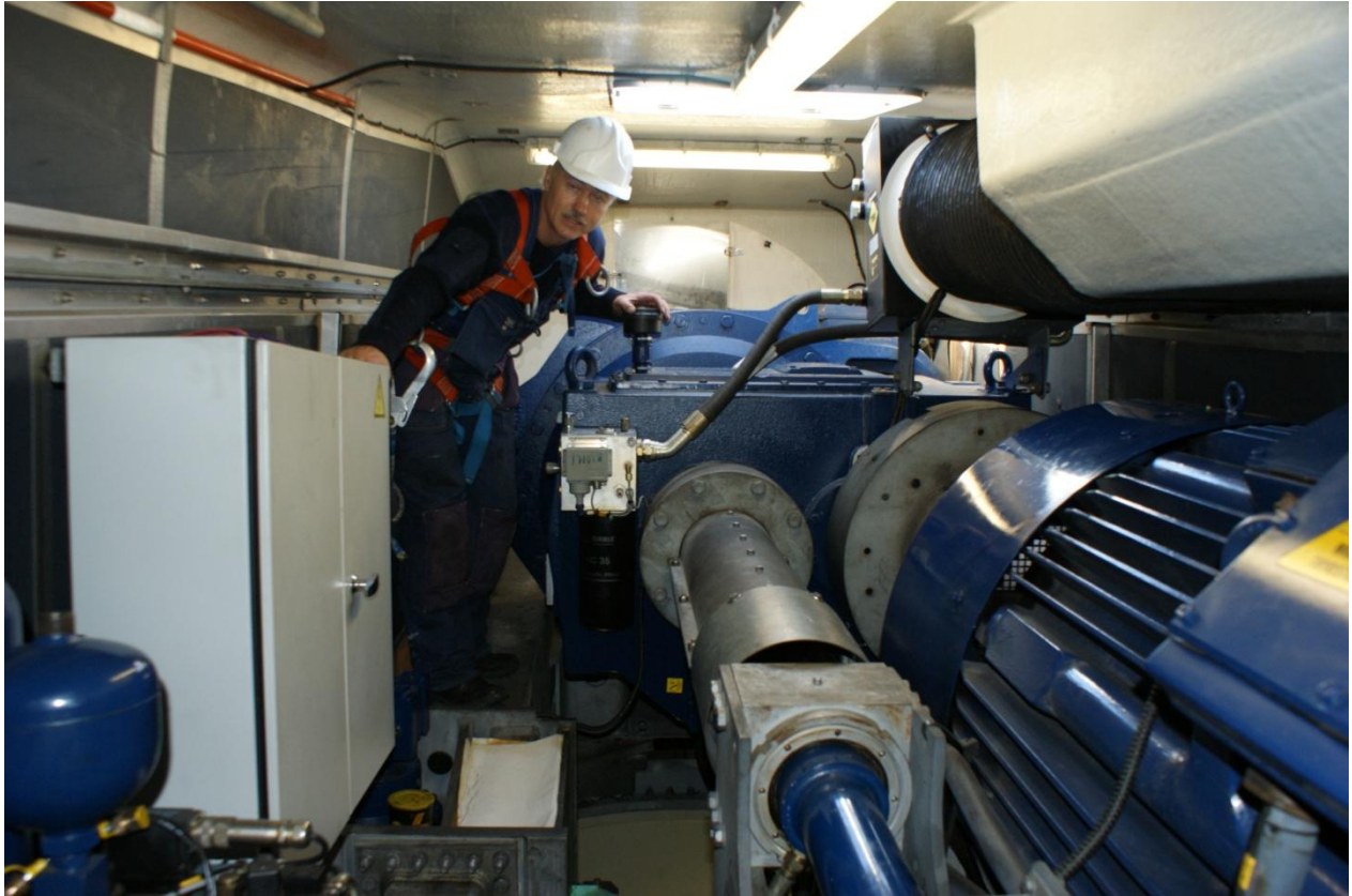
FIGURE 40: INSIDE A NACELLE. PITCH CONTROL HYDRUALIC DYLANDER IN THE MIDDLE, INDUCTION GENERATOR TO THE RIGHT.
