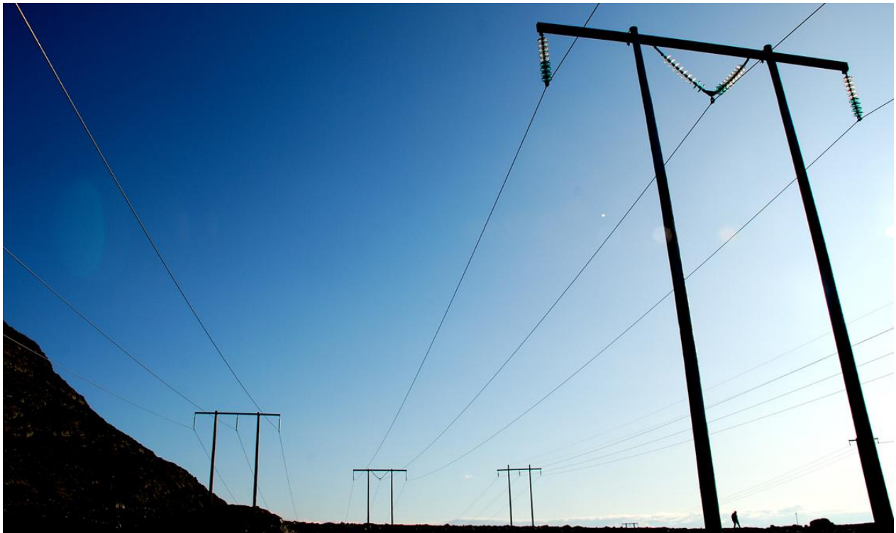
FIGURE 29: OVERHEAD LINES IN NORTHERN NORWAY.
