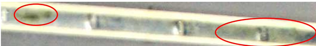
Figure 15. At 1500 hours DH-A show corrosion on the bus bars on the back of the cell.
