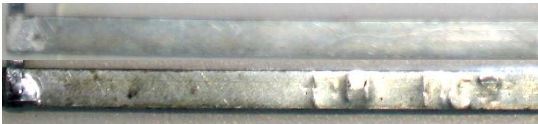
Figure 46. A small corrosion start to show on the back side of DH-B3, 1500 hours.
