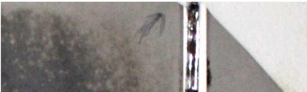
Figure 90. Discoloured back side and corrosion on the back side bus bar, DH-D5.
