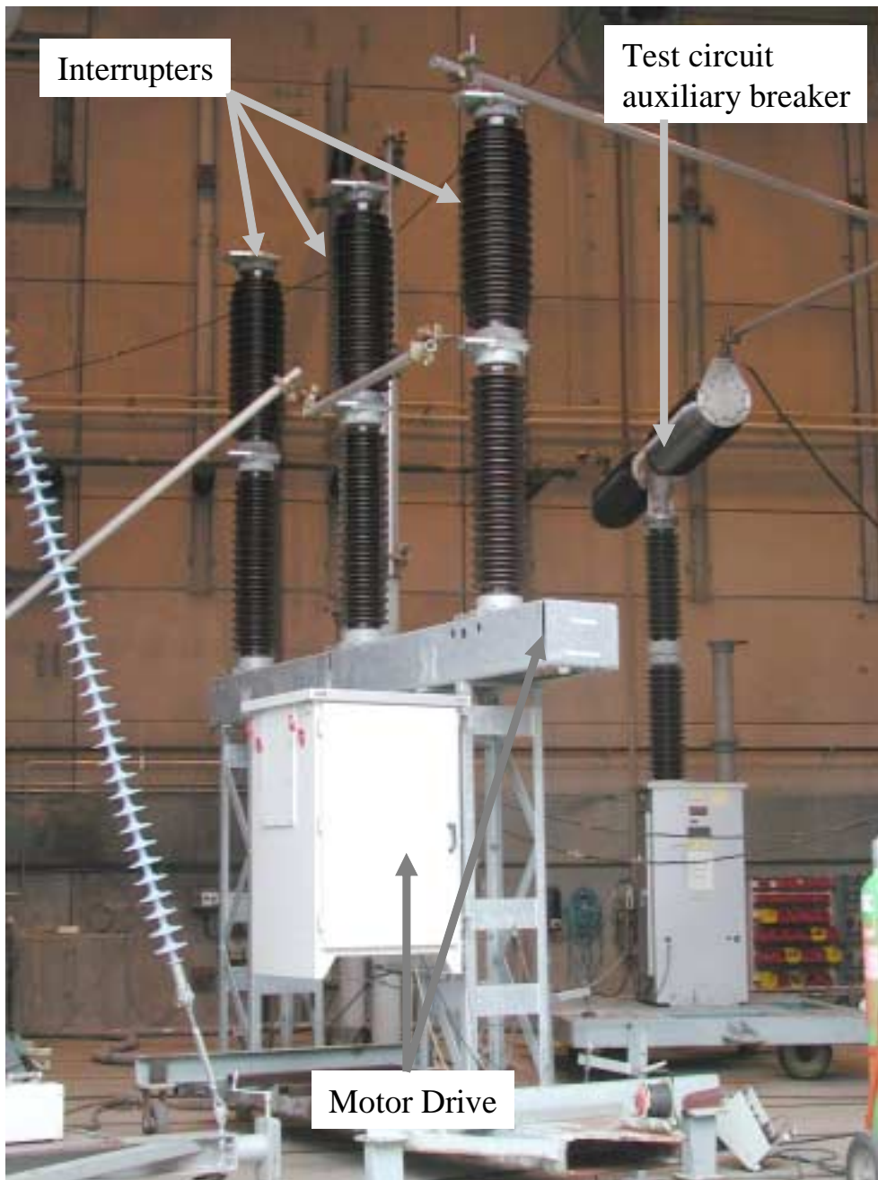
Figure 3.2: HV SF 6 circuit breaker used for high power experiments (Photo courtesy of ABB AB©)
