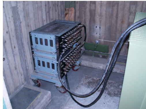
fig. 70. Photo of Resistive load ( R=0.5 \Omega )
