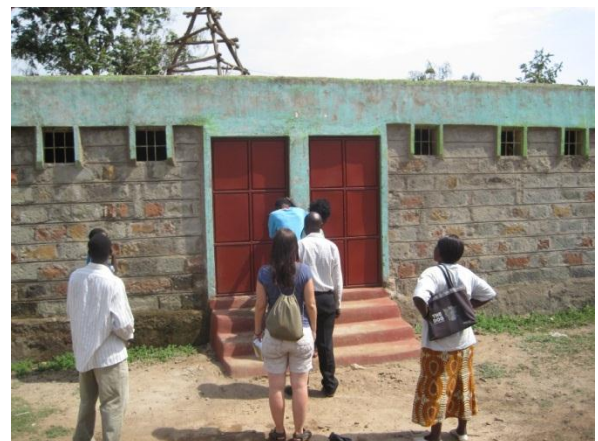
Plate 21. Picture showing a section of the Nyalenda Bio Centre under construction
