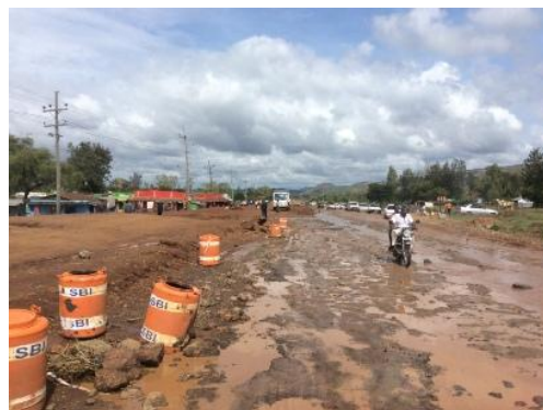
Figure 13. Kisumu-Busia road. Construction on the left, main road on the right
